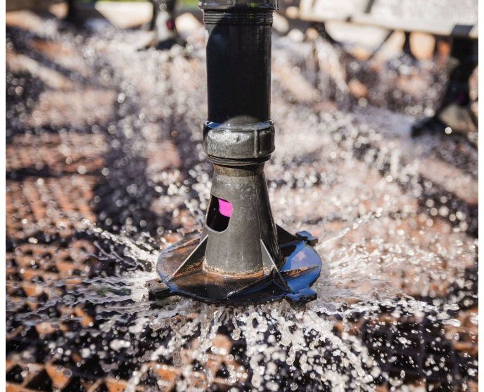
Figure 1: Clog-resistant nozzles provide even distribution of wastewater over the media
